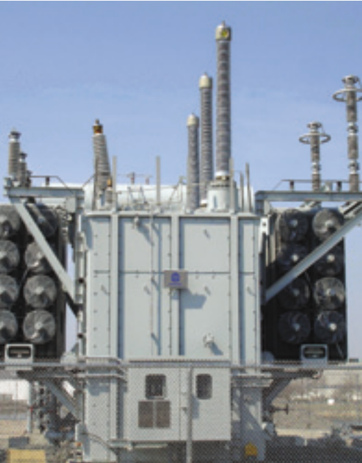
345kV Transformer
