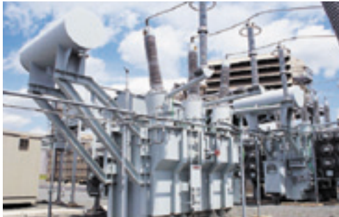
230kV Transformer
